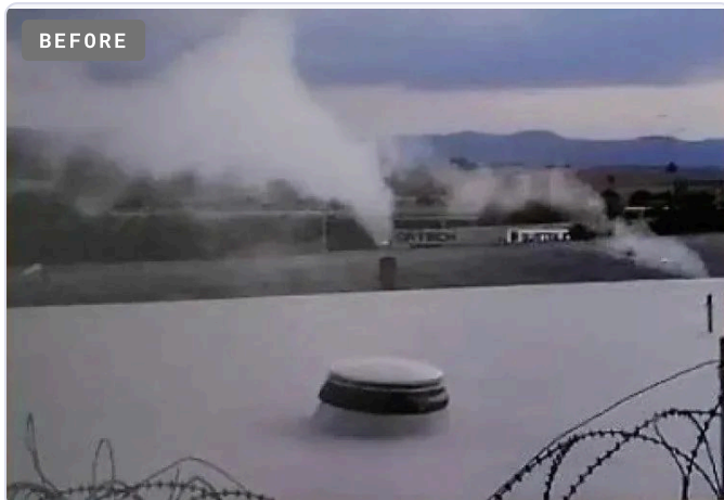
Before the retrofit: steam venting from the plant roof.
